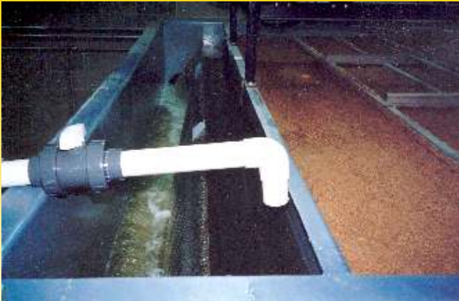
IWWS Physical/Chemical Waste Treatment System showing clean effluent overflow (left), sludge removal (center) and sludge holding compartment (right).
